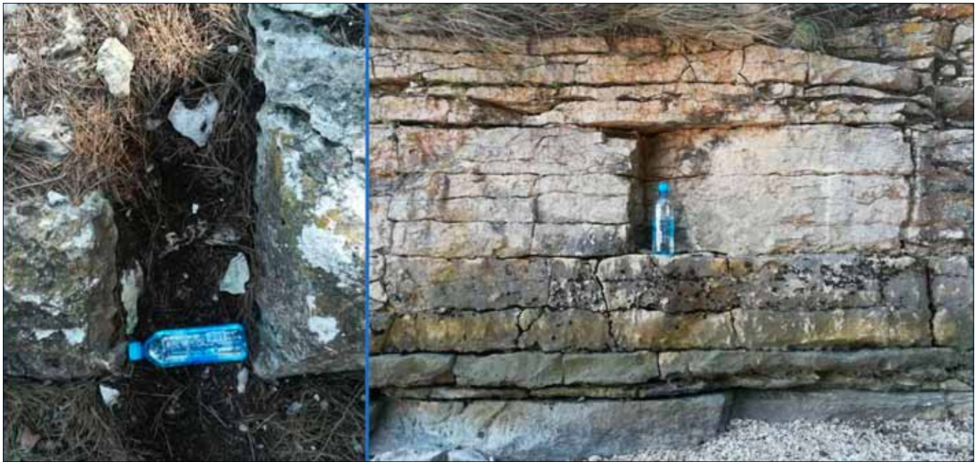
Figure 3. A quarry on Mugli Cape, Premantura: on the left side a pašarin, on the right side platy limestone. Height of the water bottle 21 cm (made by: Katarina Šprem).
