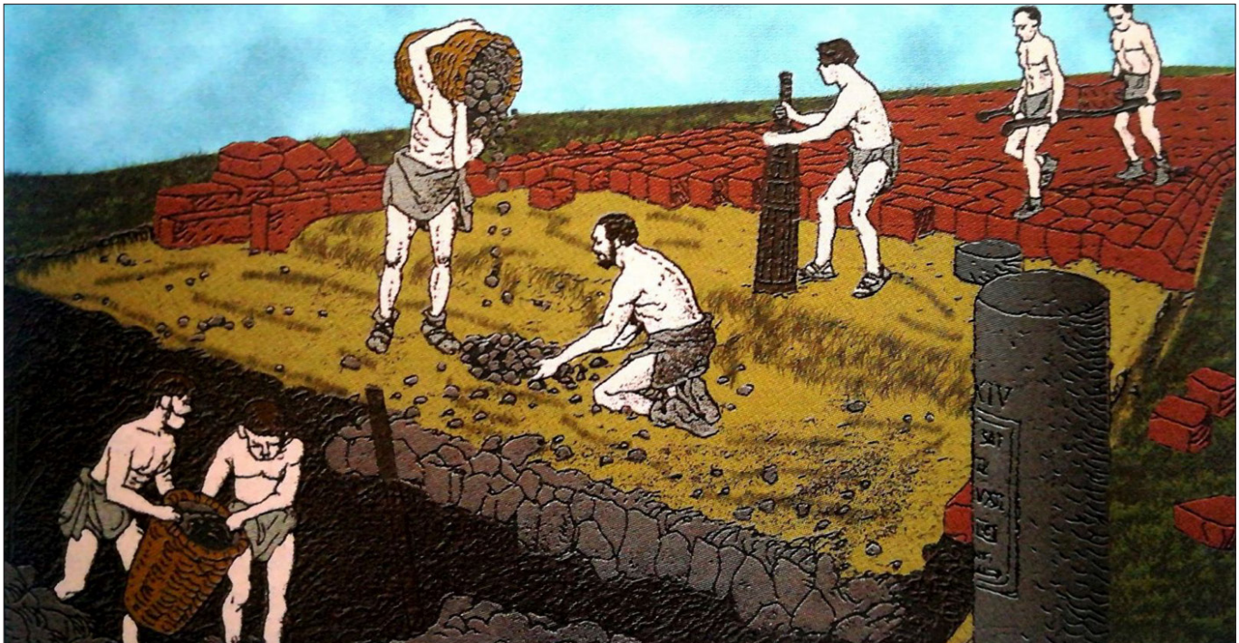
Figure 15. Road construction at different stages (after Goldstein 2007:371).
