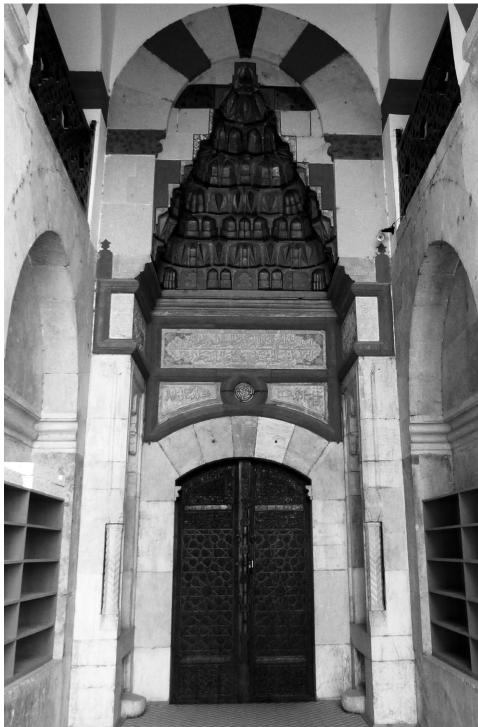
fig. 3. Bāyezīd Pasha zāwiya gate, photograph by the author
