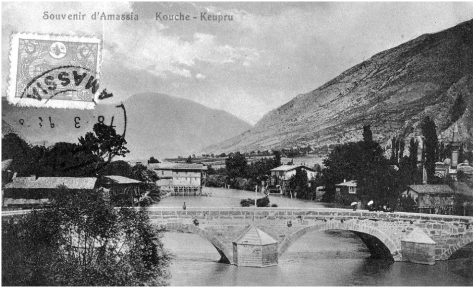
fig. 7. Hünc Bridge (Kuş Köprü) in Amasya, thirteenth century, with Bāyezīd Pasha zāwiya on the right prior to the removal of its added minaret, early twentieth century postcard, by permission of D. Loupis Visual Collection of Islamic Architecture, Athens-Greece
