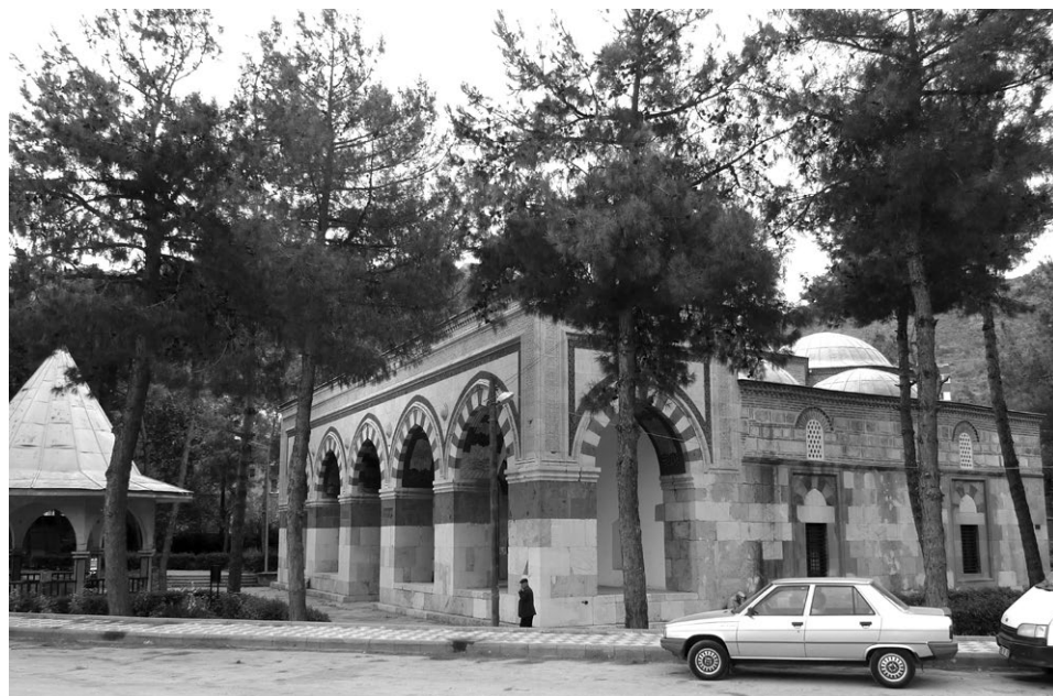
fig. 6. Bāyezīd Pasha zāwiya, general view from the road, photograph by the author
