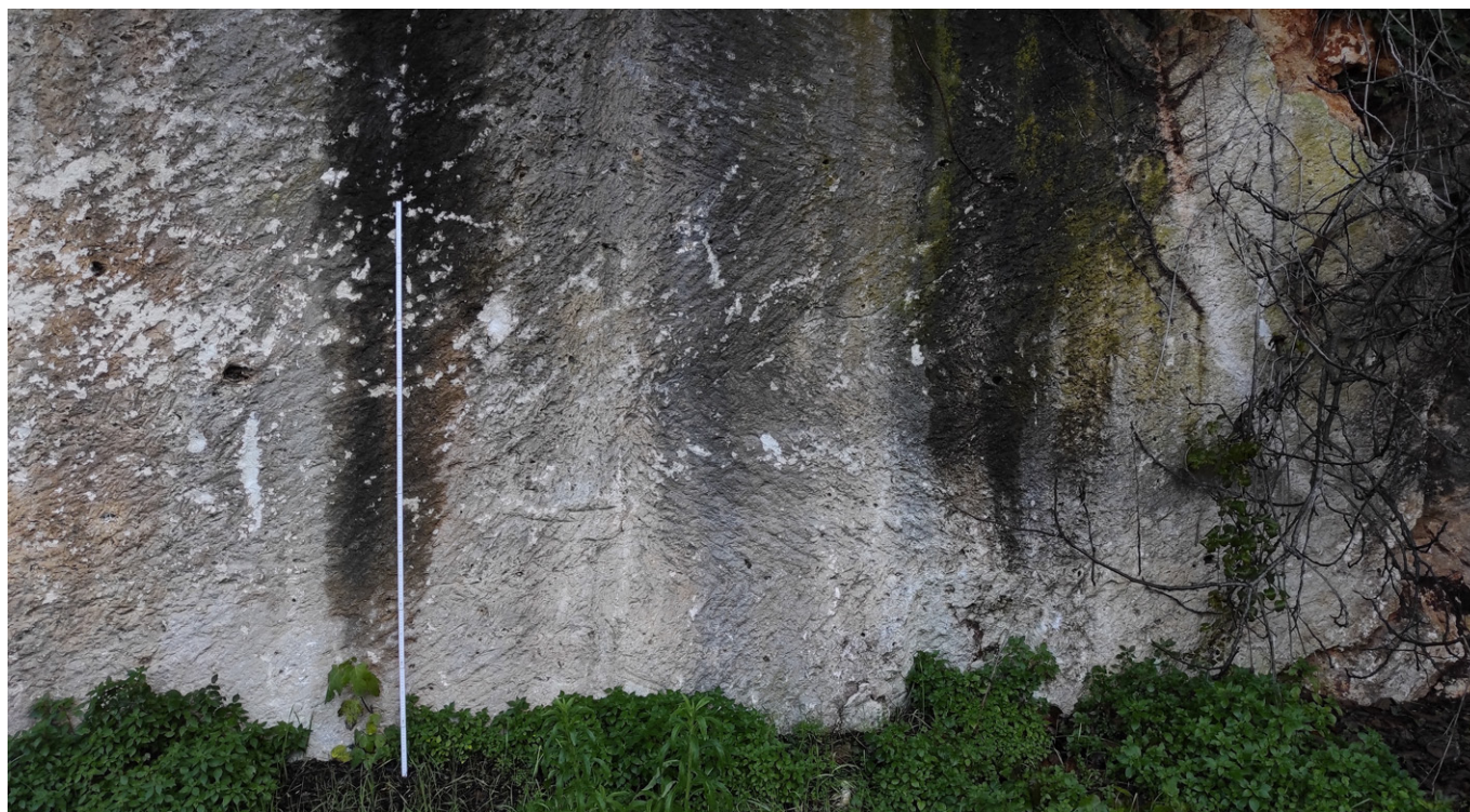
Figure 5. Tool traces on a quarry wall in the Roman part of the quarry, Cave Romane, Vinkuran. Height of the wooden meter – two meters.
