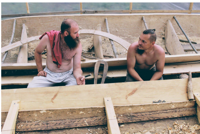
Figure 19. Repair. (Archive of the project Medieval Shipyard ).
