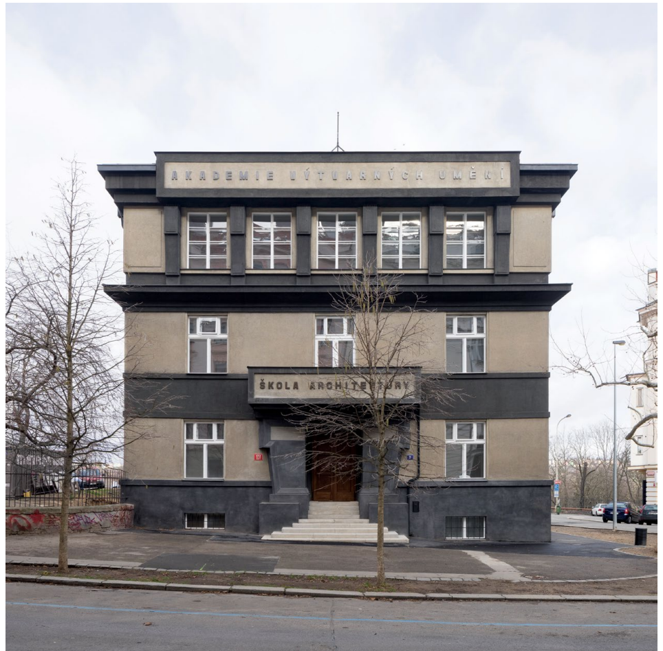
Fig. 3. Jan Kotěra and Josef Gočár, Mistrovská škola architektury (Master School of Architecture), Academy of Fine Arts, U Akademie 2, Prague, original building project 1922–1924. Renovation by Marcela Steinbachová, Skupina Architekti, 2018–2020. Photograph by Tomáš Souček.
