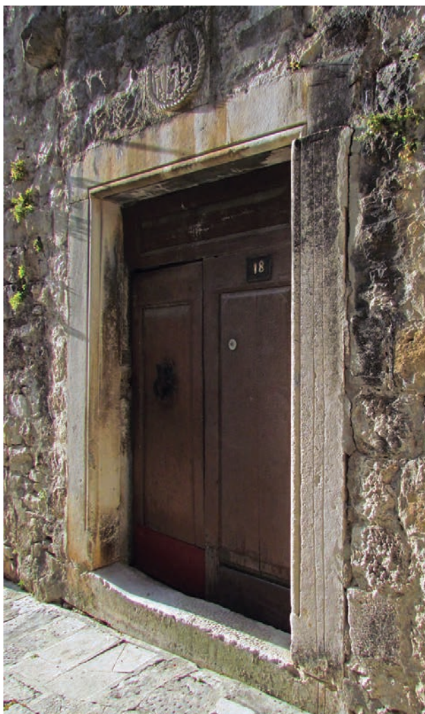
Fig. 3. Korčula. Measuring mark carved in the door jamb of the Giunio-Fisković house.
